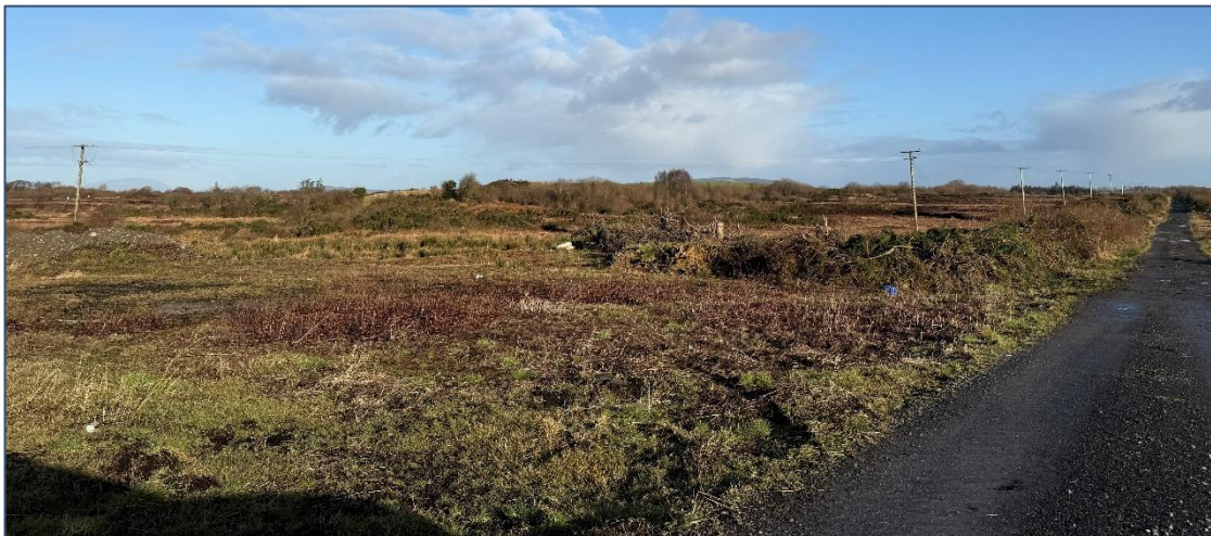
Plate 13-12 Views north-west towards the Site from the local road (L15053), approx. 380m south of turbine T4
